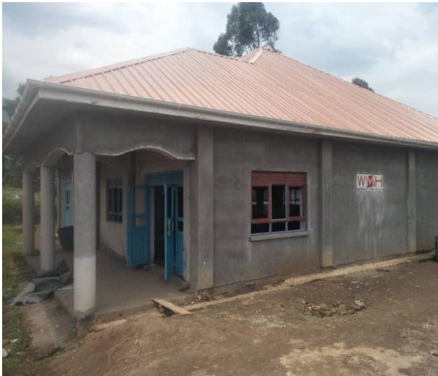
Photo: Construction of multipurpose main hall
